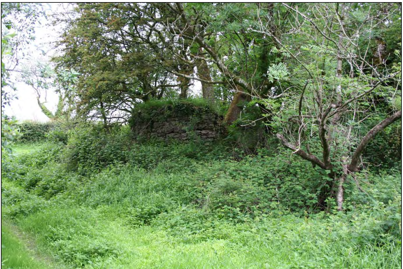
Plate 18: Limekiln (PRN 17070) immediately north-west of site, looking north
